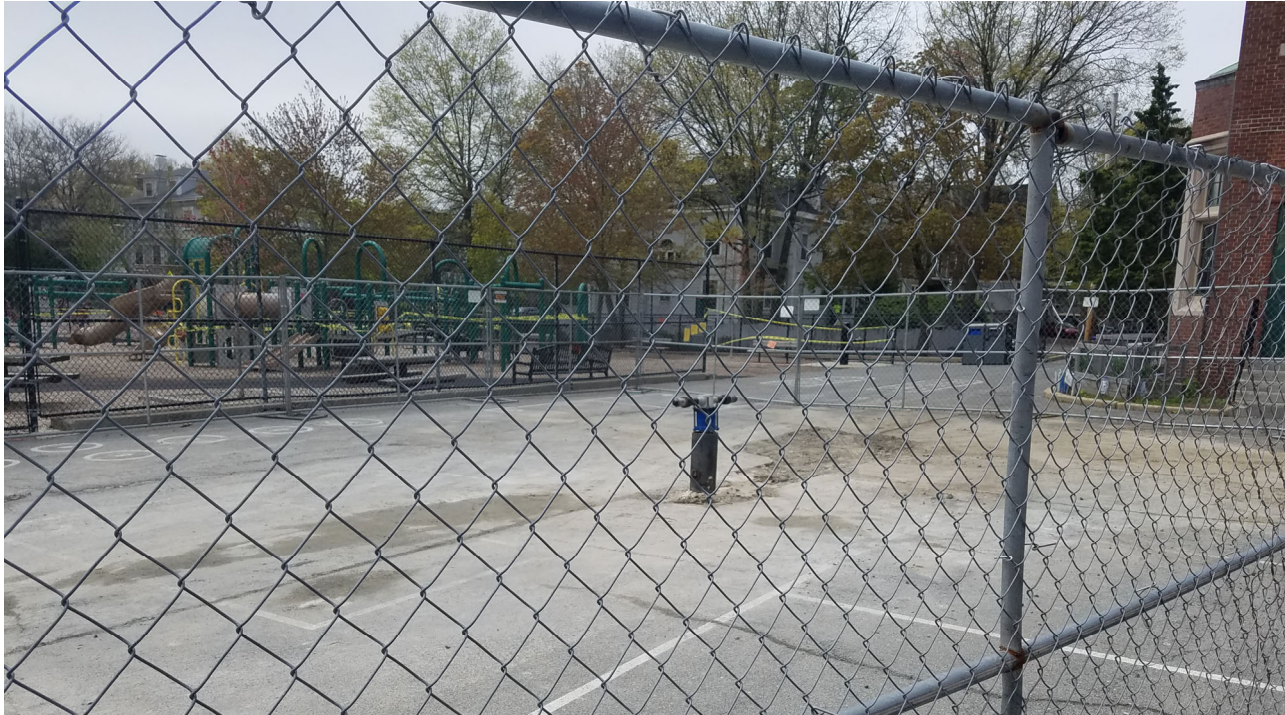
Geothermal Test Well Installed
